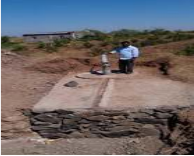
Implemented Bore Well Recharge Structures in Maharashtra (Aurangabad & Sanqli)
