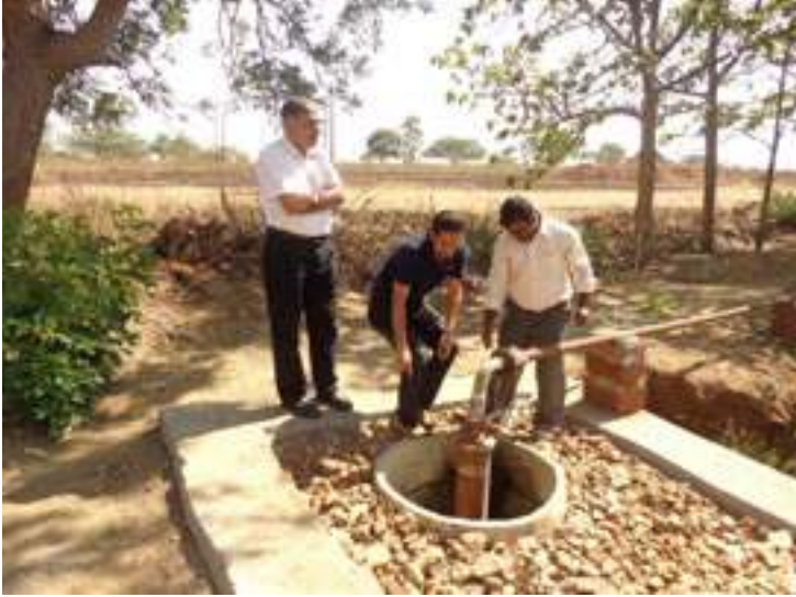
recharge implement bore well recharge ORA Hospital in Washim at Maharashtra
