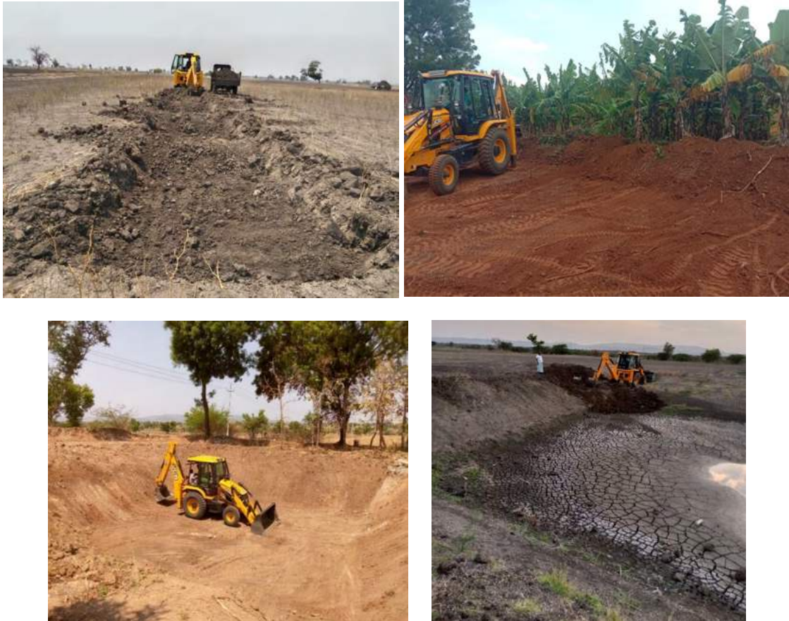
Farm pond and bund construction in progress in Peta Alur
