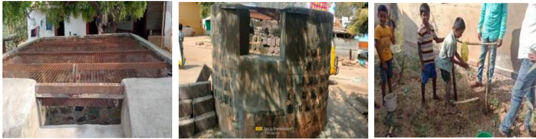
Cleaning and laying of mesh over open wells
