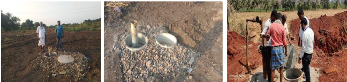
8 borewell recharges bore well recharge interventions executed in Kelur
