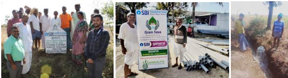
Farmers with pipes being installed in their fields for irrigation
