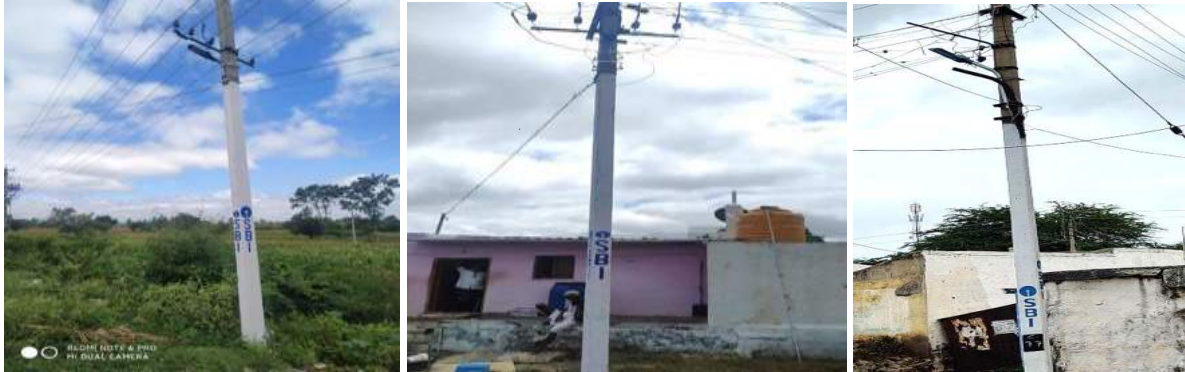
Street lights installed in the village roads
