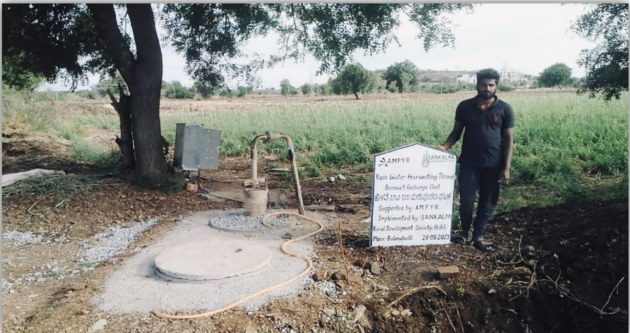
Bore well recharge system
