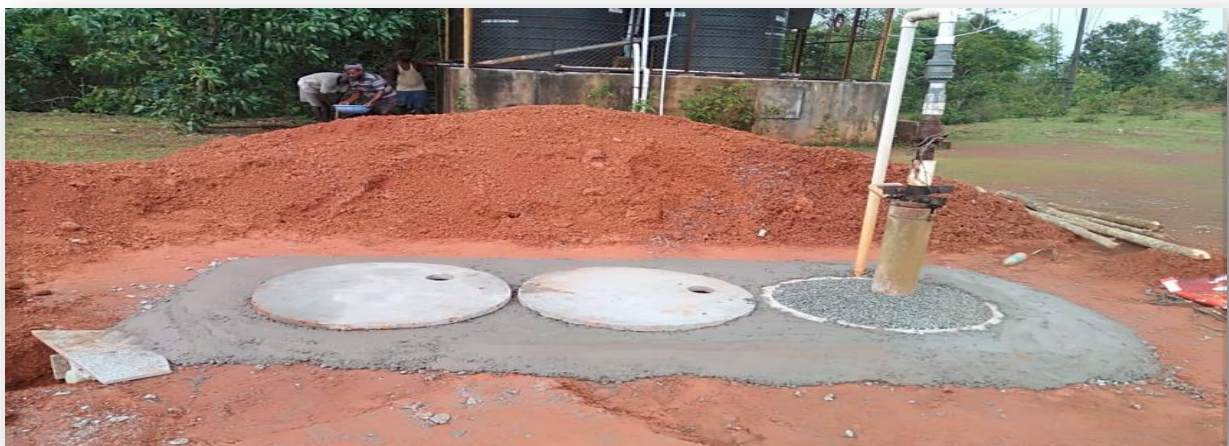
Bore well recharge system
