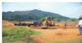
Lake desilting work in progress at Kelur village in Mundargi taluk
